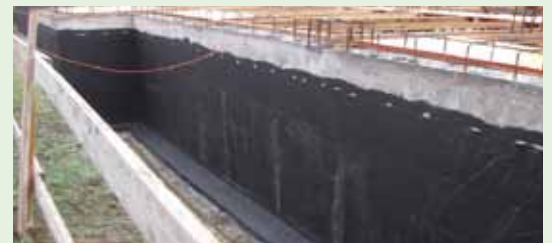
Protect the waterproofing with PROTEFON TEX or EPS panels
